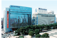
Matsuzakaya Nagoya (Floor space: 86,758 m 2 )
