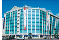
Matsuzakaya Shizuoka (Floor space: 25,452 m 2 )
