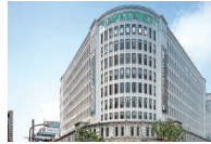
Daimaru Kobe (Floor space: 50,656 m 2 )
