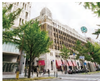
Daimaru Osaka Shinsaibashi (Floor space: 77,490m 2 )
