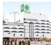
Shimonoseki Daimaru (Floor space: 23,912m 2 )
