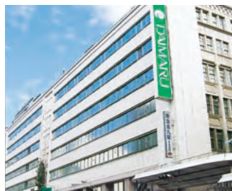
Daimaru Kyoto (Floor space: 50,830m 2 )
