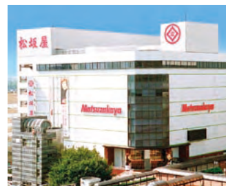
Matsuzakaya Toyota (Floor space: 18,220m 2 )
