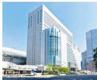
Daimaru Osaka Umeda (Floor space: 64,000m 2 )
