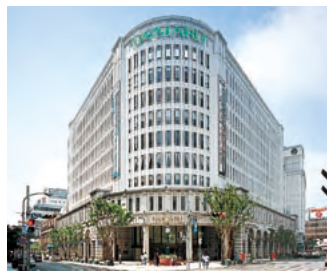
Daimaru Kobe (Floor space: 50,656m 2 )
